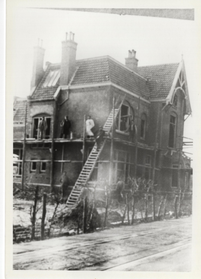
Unknown building in Amsterdam by G.J. Roozee. He is the one on the ladder
